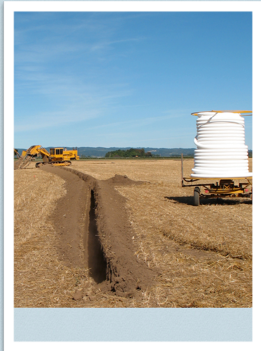
Field Tiling being installed in trenches Photo by Cherry Amabisca
